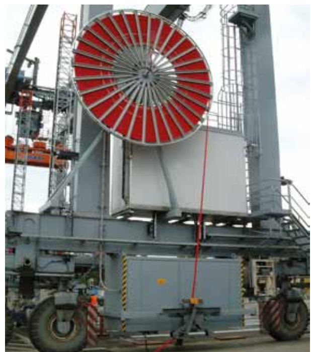
Motor cable reel in RTG operation
